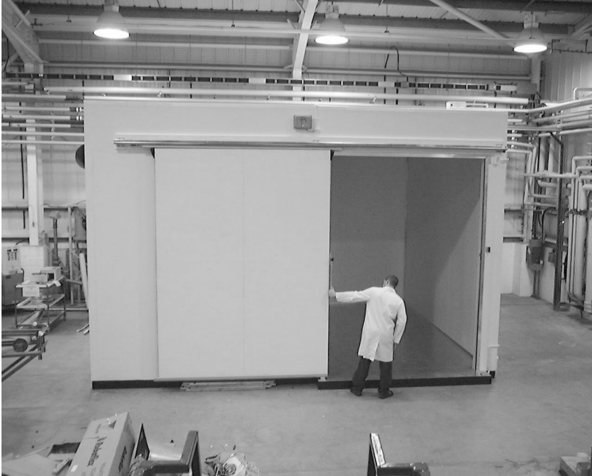
Figure 1. Cold store with a large single opening constructed inside a processing hall at FRPERC, University of Bristol.
