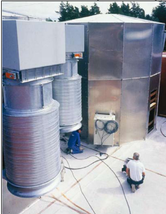
Photo 4.1: Phase reactor magnetic field shielding (on right hand side), applicable to a STATCOM installation
