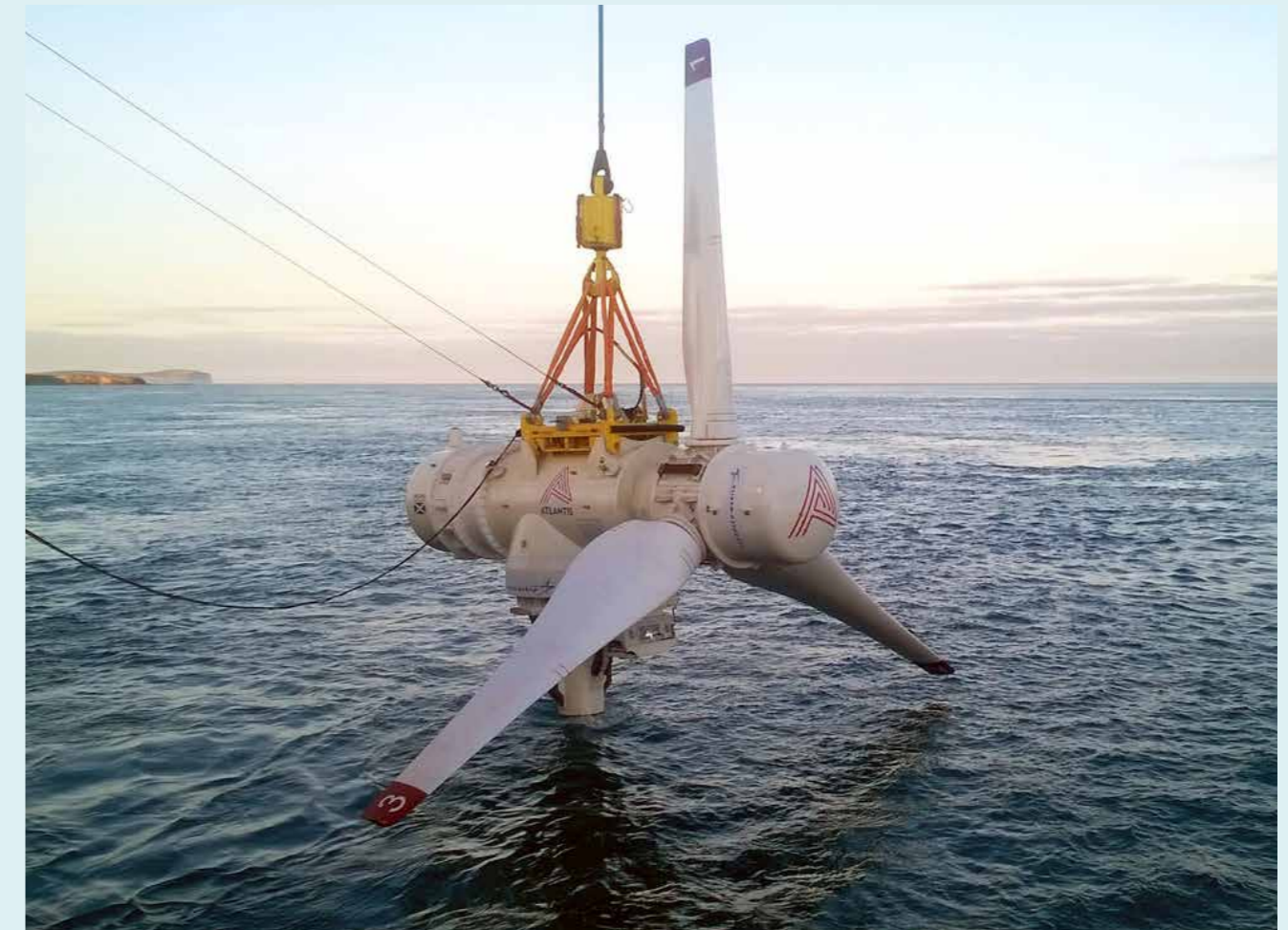
AR1500 tidal turbine being deployed at MeyGen (Credit: SIMEC Atlantis)
