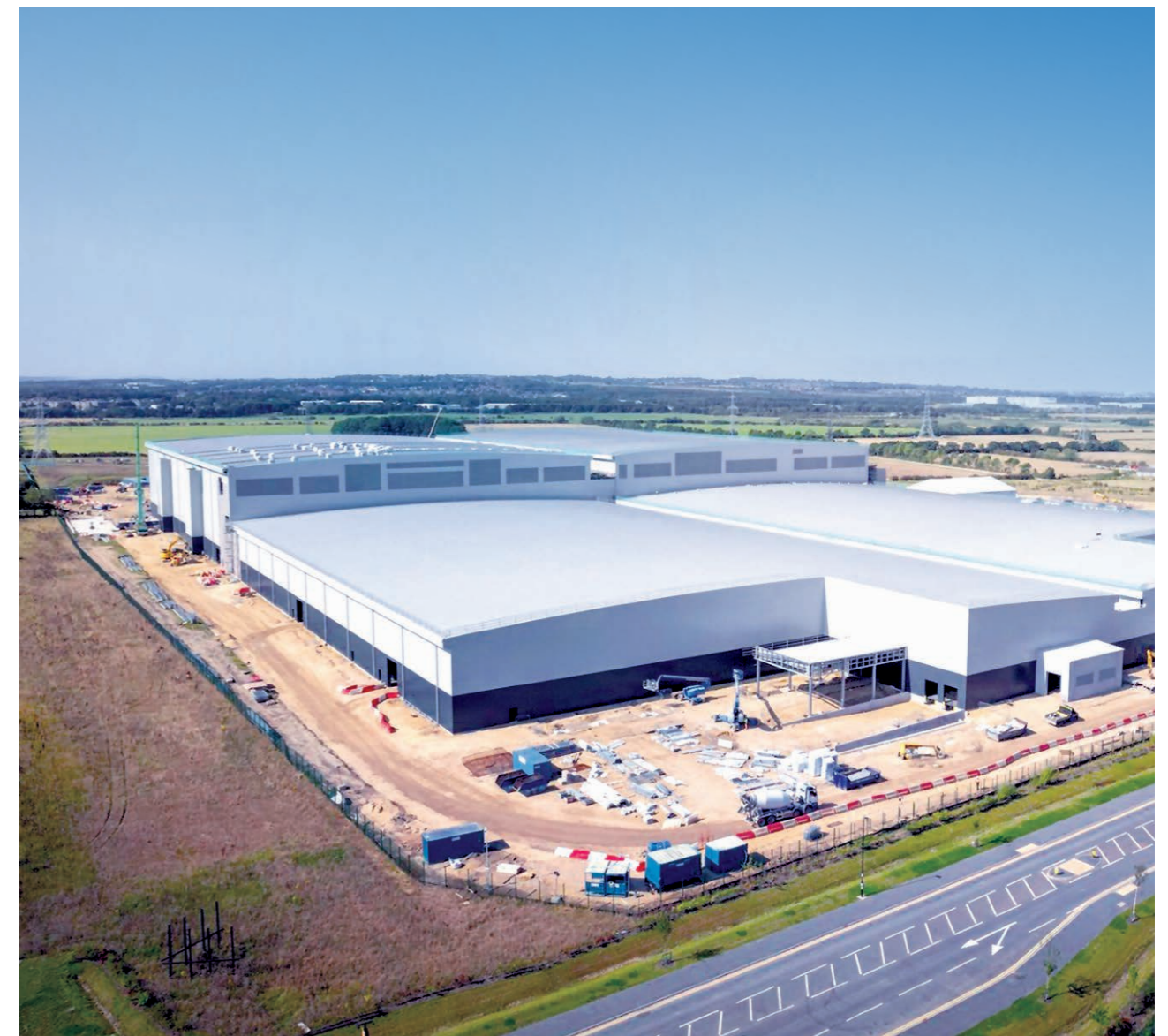
AESC gigafactory under construction, Sunderland
