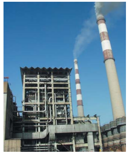
Figure 2. Yaomeng Unit No.1 before Refurbishment
