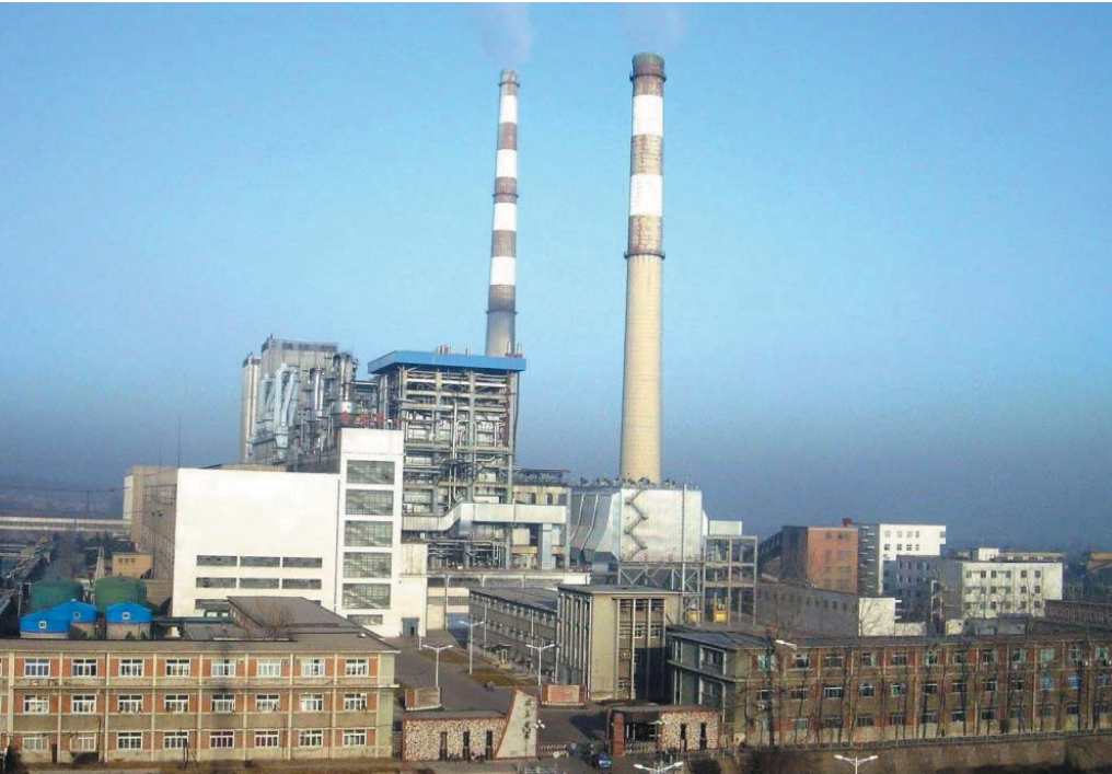
Figure 1. Yaomeng Boiler No. 1 as it is today
