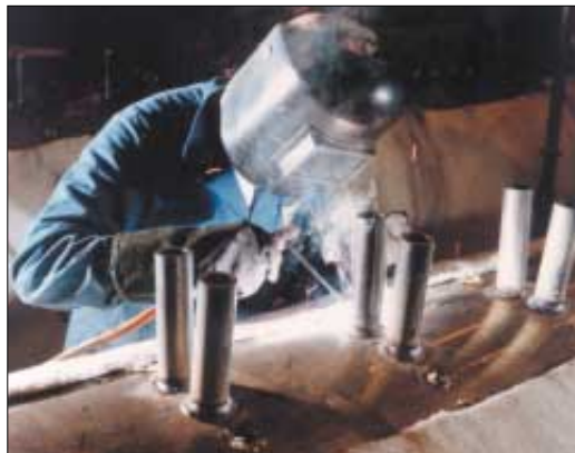
Manual metal arc welding of advanced steel
