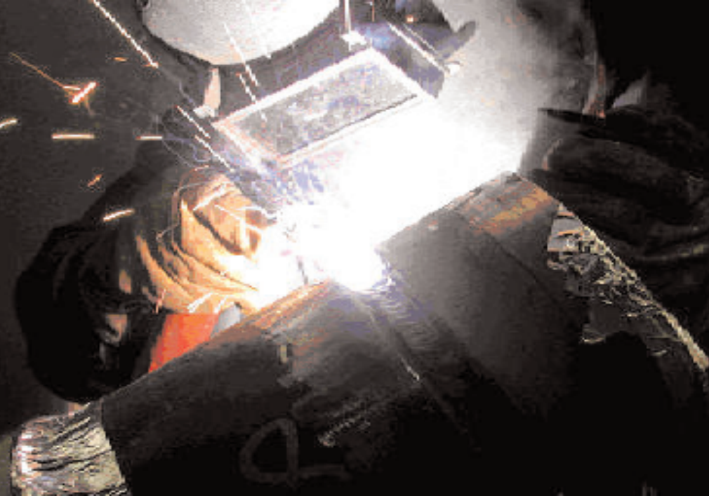
Figure 1. MMA welding in the 45° inclined position (courtesy of MBEL)
