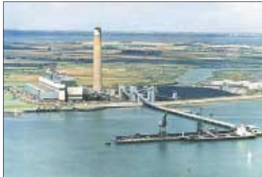
Kingsnorth Power Station – site used for full-scale plant trials
