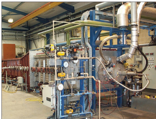
Innogy's 0.5MW Combustion Test Facility on which experimental tests will be carried out during the project
