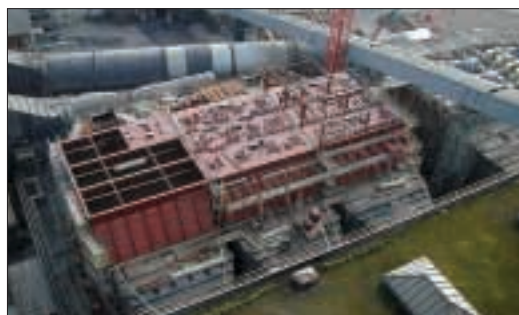
Construction of precipitators on a 500MWe generating unit
