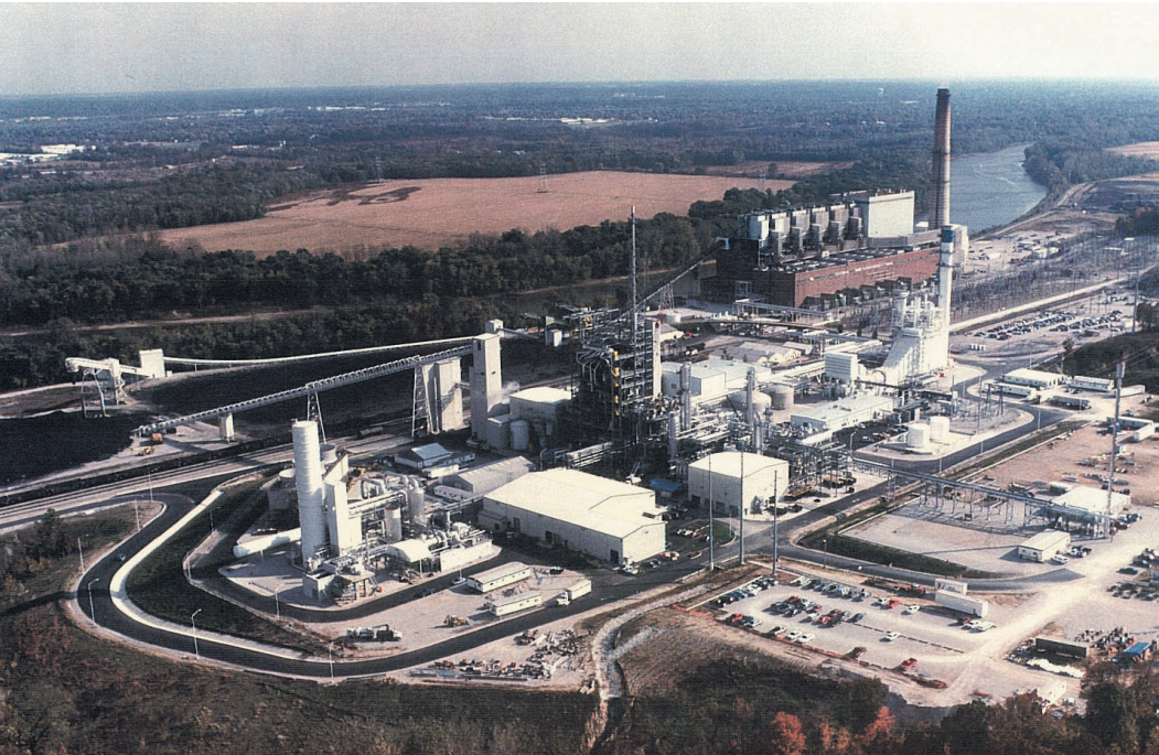
Wabash Coal Gasification Plant in Indiana USA
