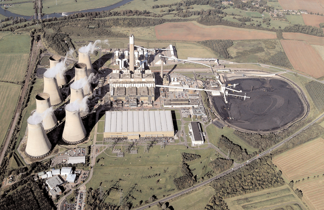
Figure 1. Ratcliffe Power Station (4 x 500MWe Sets), UK, E.ON UK
