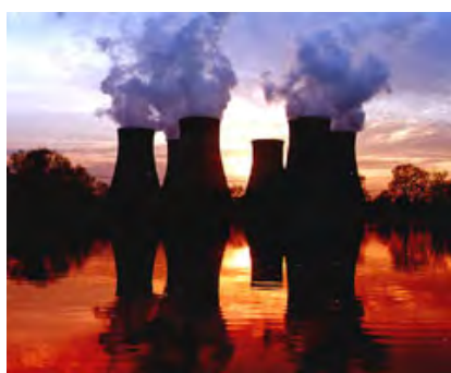
Figure 2.1-2: Drax Power Station
