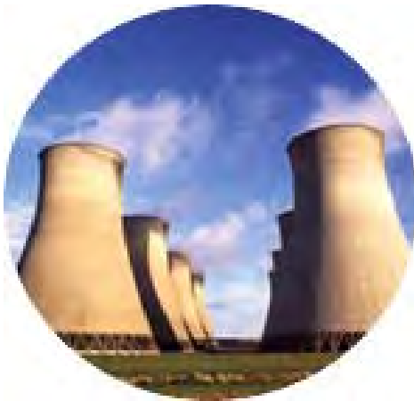
Figure 2.1-3: West Burton Power Station
