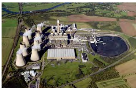
Figure 2.1-1: Ratcliffe Power Station
