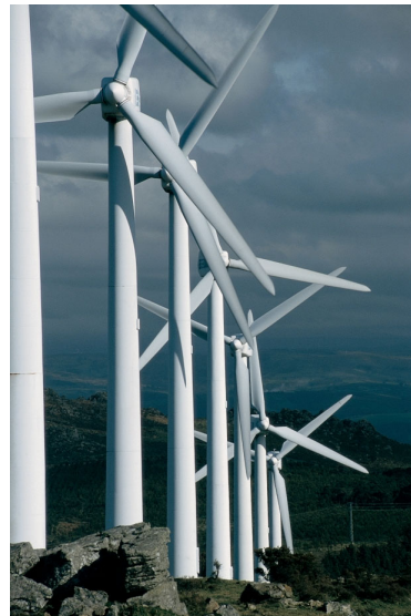
Demanding conditions for wind turbines on a Spanish hillside (courtesy of LM Glasfiber A/S)
