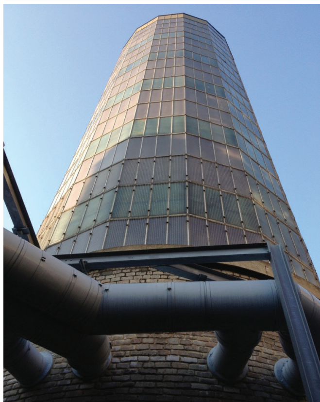
Figure 22. The Thermal Storage Tower has architectural appeal
