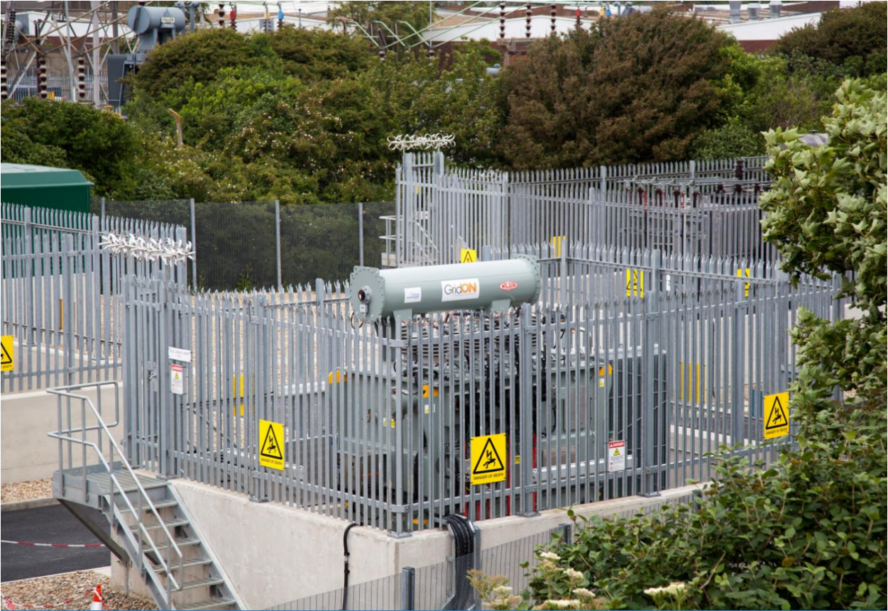
Figure 4 - PCFCL installed in the Newhaven Town substation
