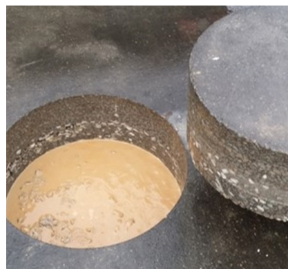
↑ Figure L: Removal of the core (Source: Tracto Technik)
