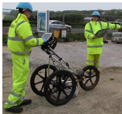
↑ Figure N: Undertaking ground penetrating radar survey
