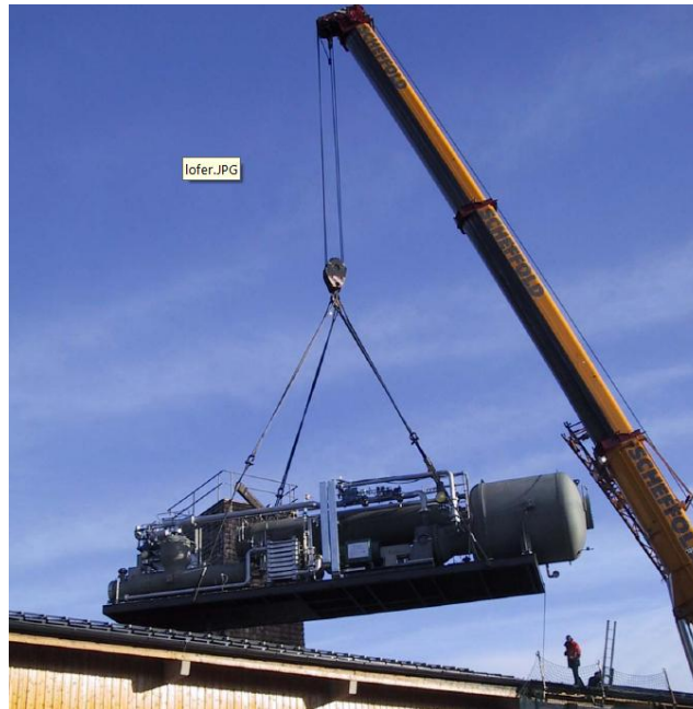
Figure 32-5 Typical single skid 700 kWe ORC unit for biomass cogeneration by Turboden (Bini, 2010).
