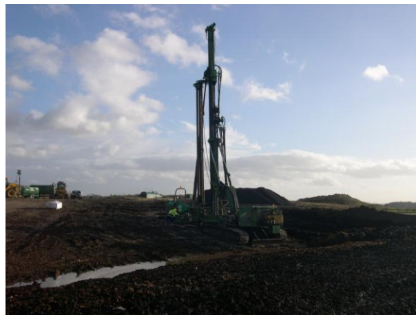
Figure 11-2 Drilling of gas extraction wells
