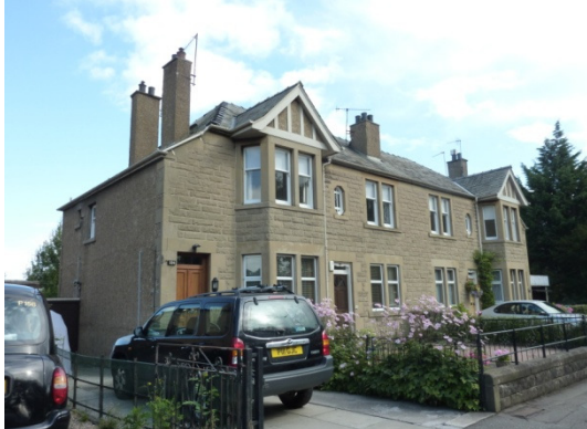
Semi-detached flats using reconstituted stone ('Forticrete'). post-1980.
