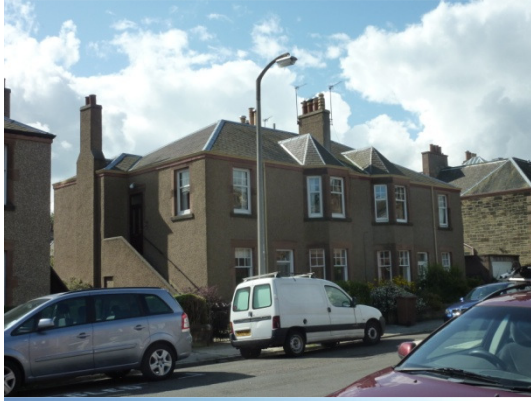
Postwar four-in-a-block house example, built en-masse to provide affordable housing after the war. Note bay window and lack of eaves depth. Also added complication of four different tenants/owners, two of whom own the first floor and roof and the other two owning the ground floor.
