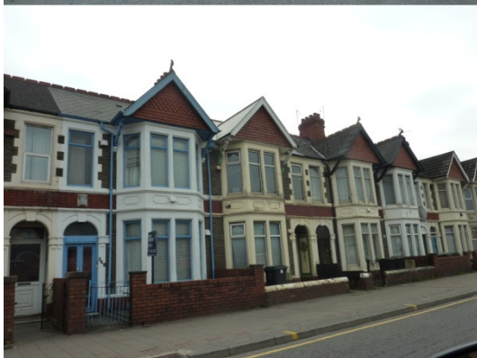
Cardiff pre-1919 terraced housing - the recessed doorways are quite a common feature, making heat loss from exposed soffits an issue.
