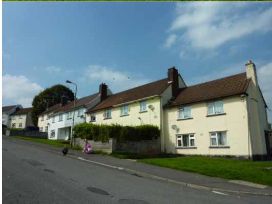
Terraced houses on a hill, showing semi-exposed party walls which may prove tricky to externally insulate. This staggered terracing is common in Wales, where the landscape in the valleys tends to be quite hilly and undulating.
