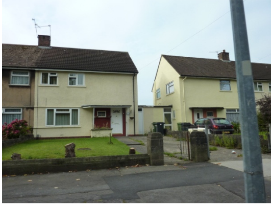
These connected sheds were a common feature for this group of semi-detached properties in Cardiff
