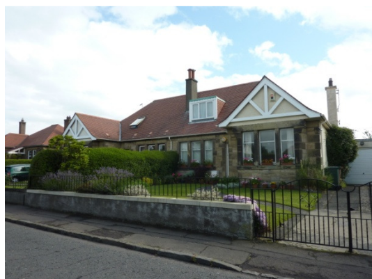
Pre-war solid stone detached house. Note use of roof ventilators and room-in-roof. Ground floor level air bricks indicate presence of suspended floor.
