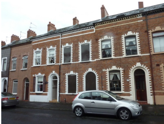
Draught lobbies are a very common feature in terraced housing. The outer door is usually non-thermal, with the inner door being the main, draughtproofed door. The outer doors are often left open in the summer and mid-season to signal a welcome to friends to come in for tea. These properties have insufficient eaves depth to install EWI without an eaves extender.
