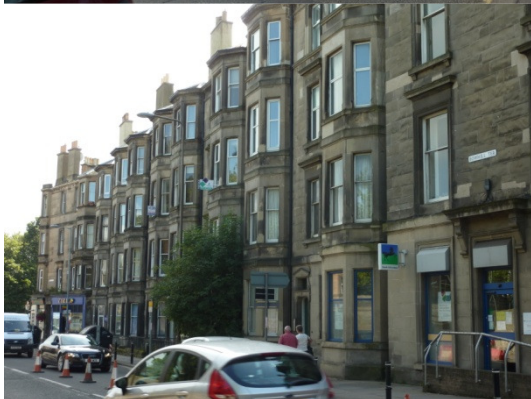
Pre-1919 Edinburgh tenement blocks - solid stone construction, full height bay windows. Often have retail on the ground floor. Likely to have highly decorated interiors. Bowhill Terrace.
