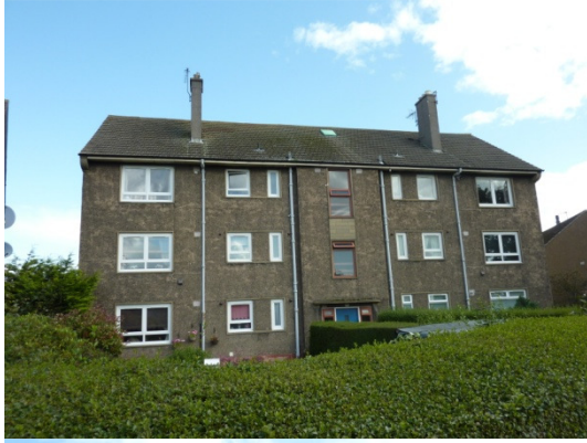
1950s low-rise block of flats. Could not see any evidence of roof ventilation features, could be an indication that no roof insulation has been installed (ventilators are a requirement when roof insulation is undertaken). Prime candidate for EWI installation.
