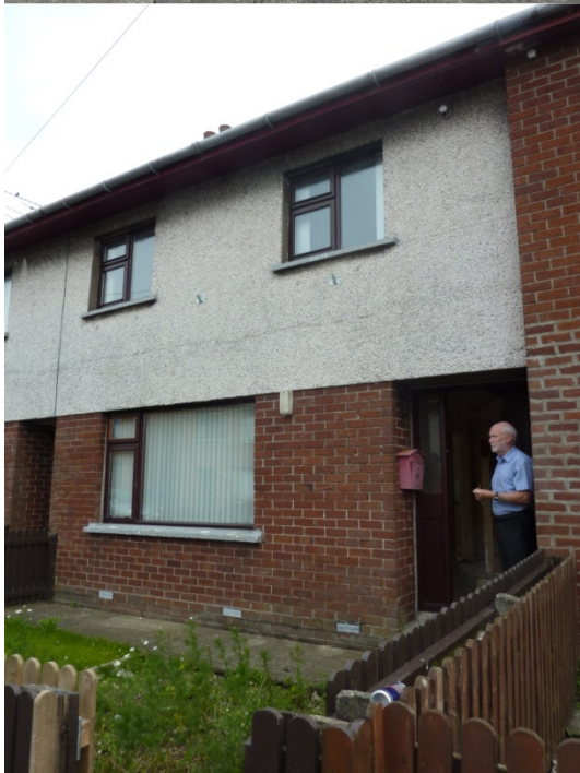
Typical Ballycastle mid-terrace property, cavity walled construction
