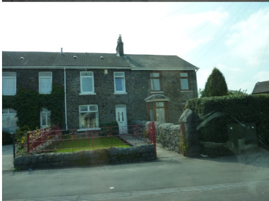
Pre-1919 stone terraced housing. The stonework here is very different from stone-built houses in Scotland, as the stone is irregular and usually a by-product of the mining industry.
