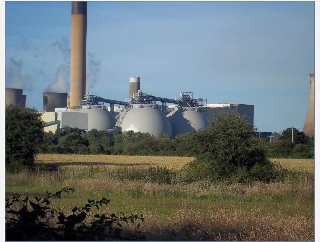
Drax - Site (showing new biomass storage area)
