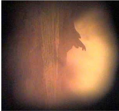
Figure 2.6 View from an 'oil burner' video probe prototype (note the slag eyebrow on the adjacent burner).
