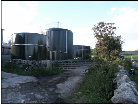
Figure 7. Farm Biogas Plant
