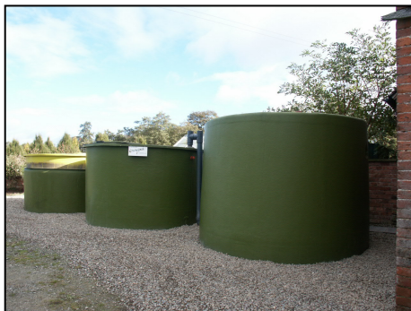
Figure 5. 20m 3 Biogas Plant
