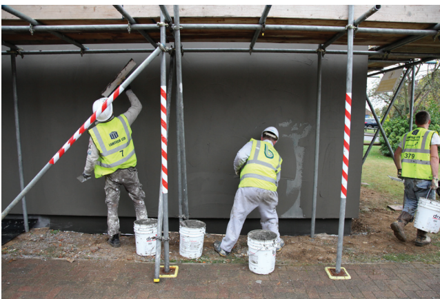
Figures 20 and 21. Resident engagement and retrofit work.
