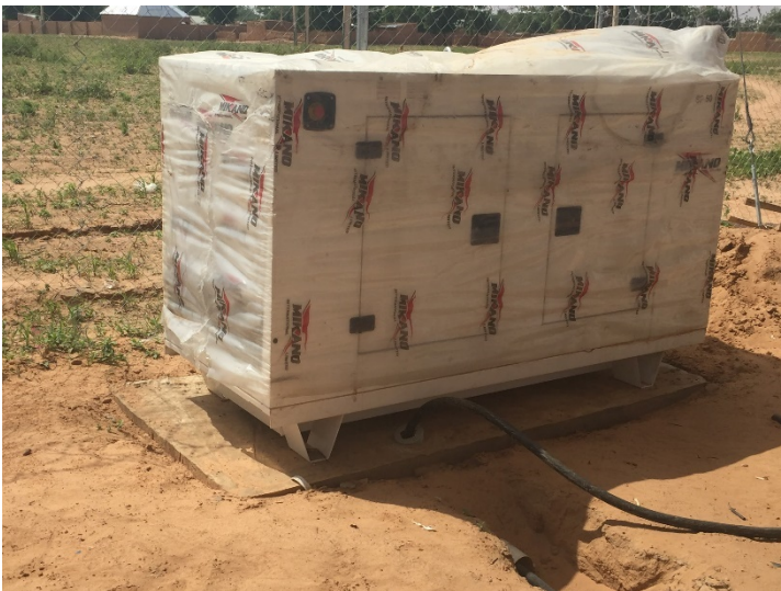
Figure 54: An example of a generator waiting installation for a rural mini grid
