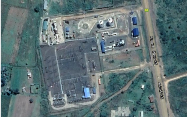
Figure 53: The site of Aggreko's 'emergency power' plant in Western Kenya
