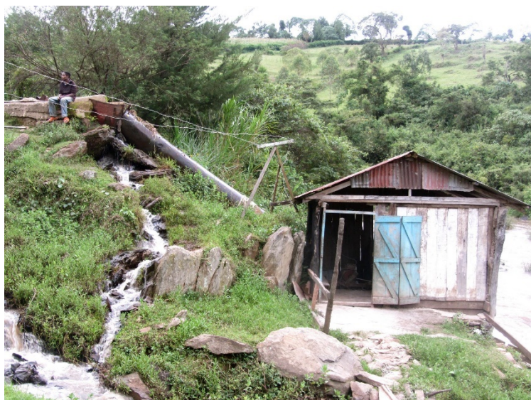
Figure 67: Kenyan micro-hydro system powering a school, a few shops, and a few homes
